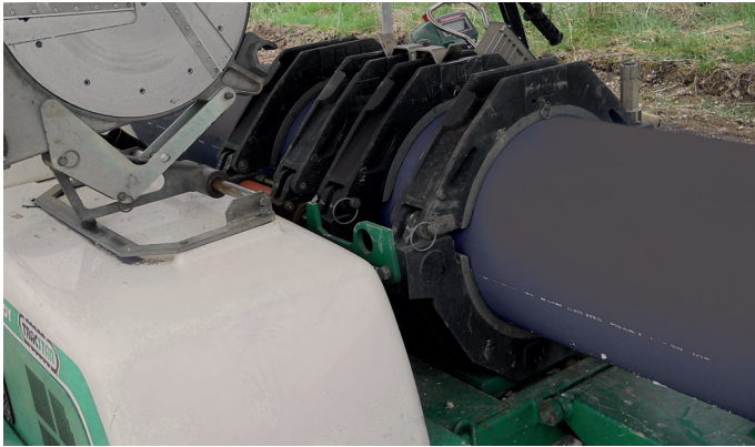
Butt-welding machine before starting the welding process
