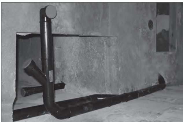
Illustration 9.2 Prefabricated pipe sections installed on site
